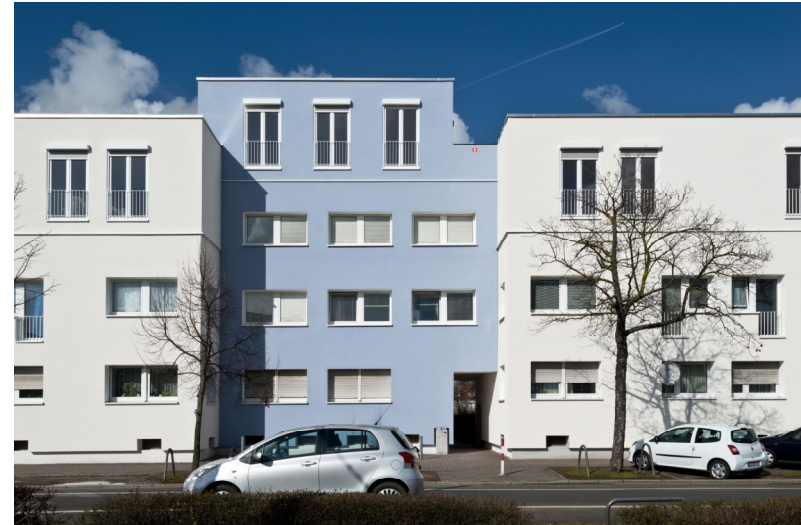
Addition of new floor plus modernization investment
