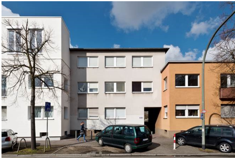
Addition of new floor plus modernization investment
