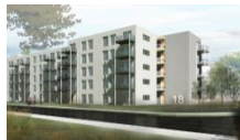
Am Ziegelanger, Landsberg am Lech 40 units, 5 floors 2,758 sqm living space €4.96m invest
