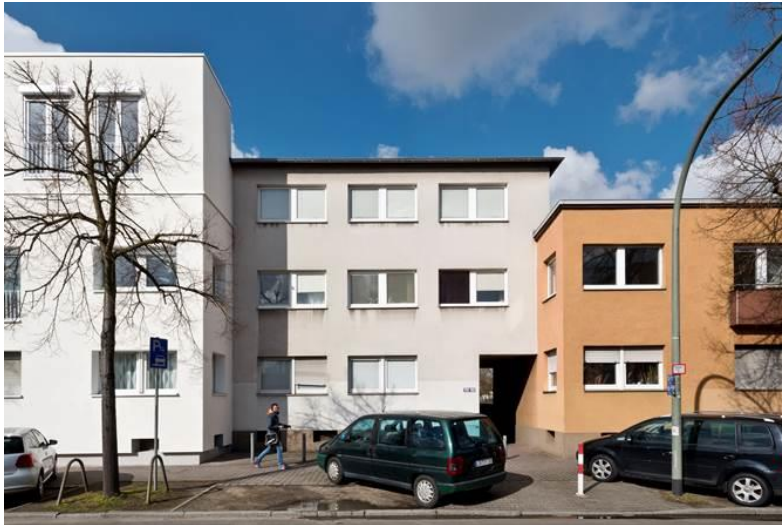
Addition of new floor plus modernization investment
