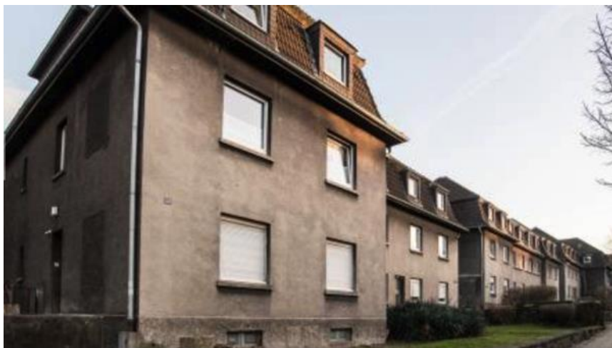
Upgrade Building - Before
