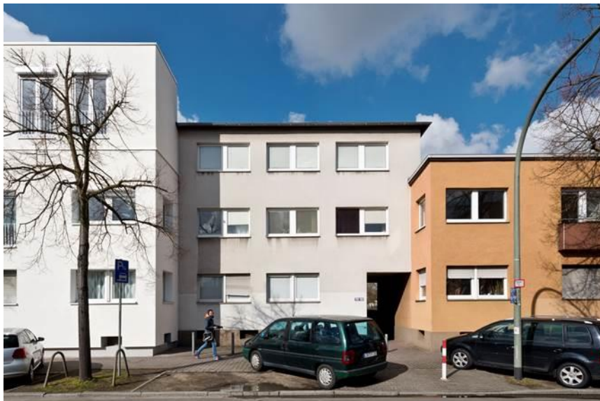
Addition of new floor plus modernization investment - Before
