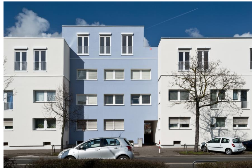
Addition of new floor plus modernization investment - After
