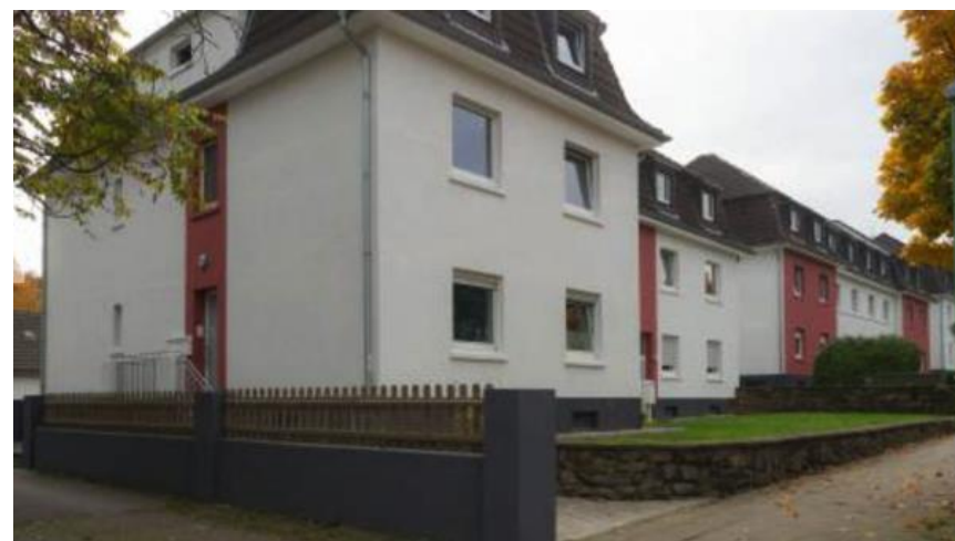
Upgrade Building - After
