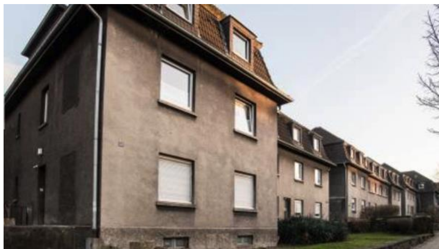
Upgrade Building - Before
