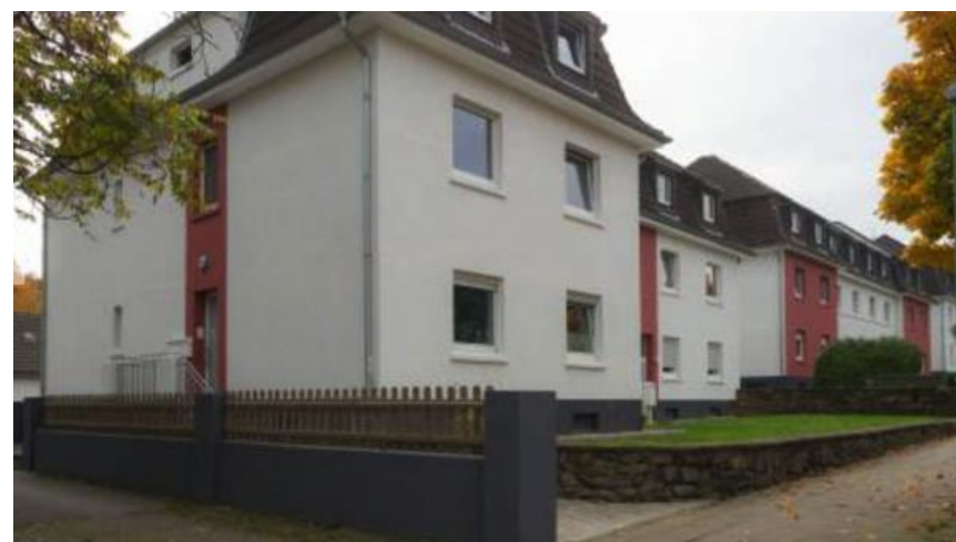
Upgrade Building - After
