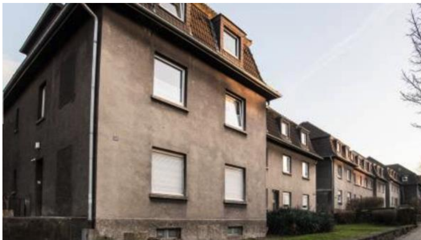
Upgrade Building - Before
