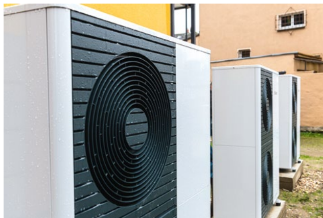
As a first step in the operational implementation, a batch of single-energy-source heat pump systems was ordered in the reporting year at short notice. Unlike the hybrid solutions often used, these run completely on electricity.
