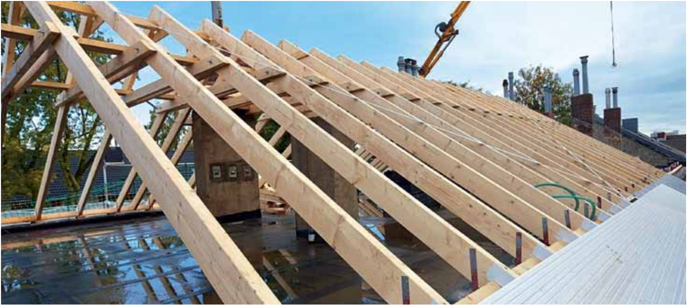
Really thorough refurbishment extends from dry foundations to a well-insulated roof.
