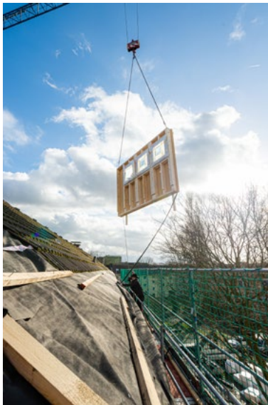
Bochum-Mitte: A series-produced Energiesprong element being carried onto the construction site.
