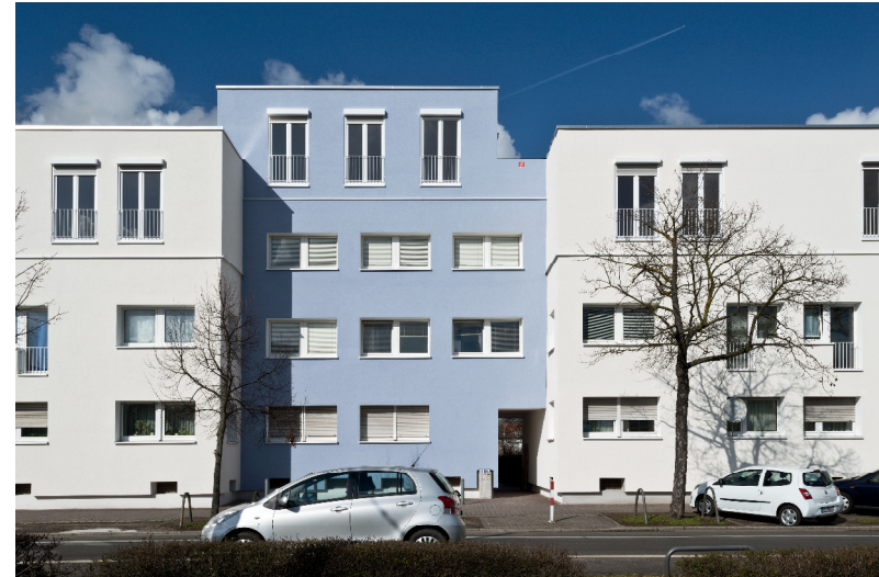
Addition of new floor plus modernization investment
