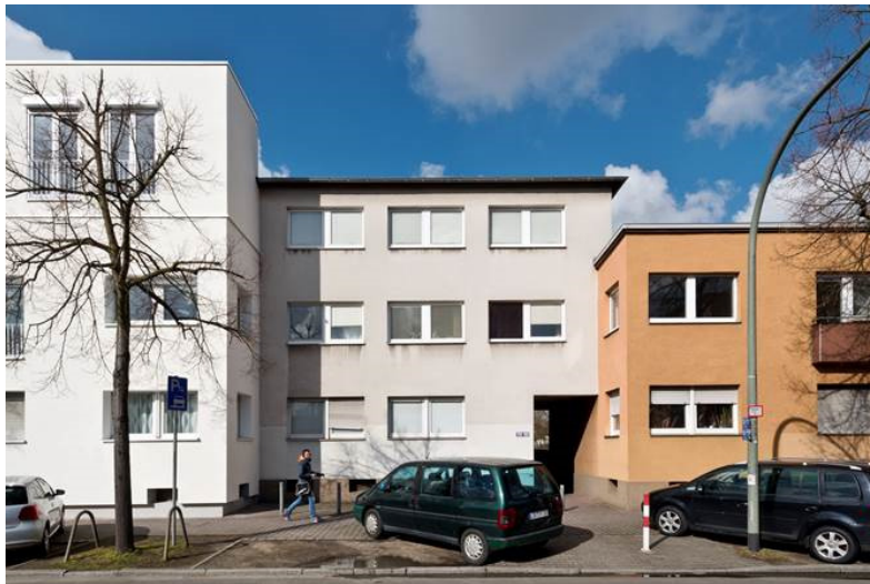
Addition of new floor plus modernization investment
