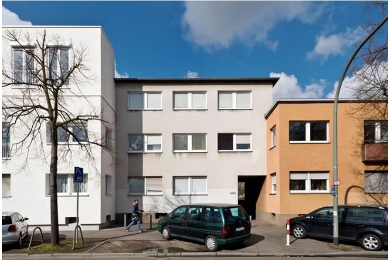
Addition of new floor plus modernization investment
