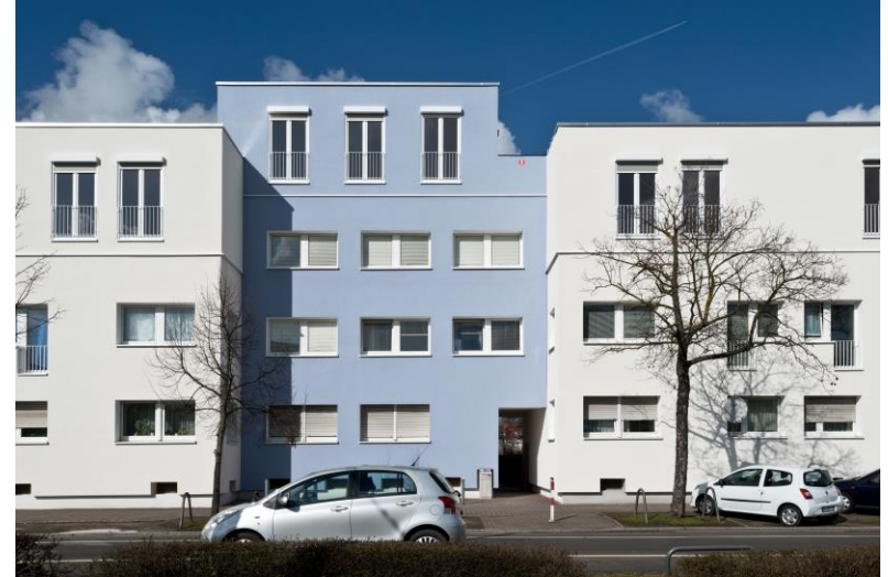
Addition of new floor plus modernization investment
