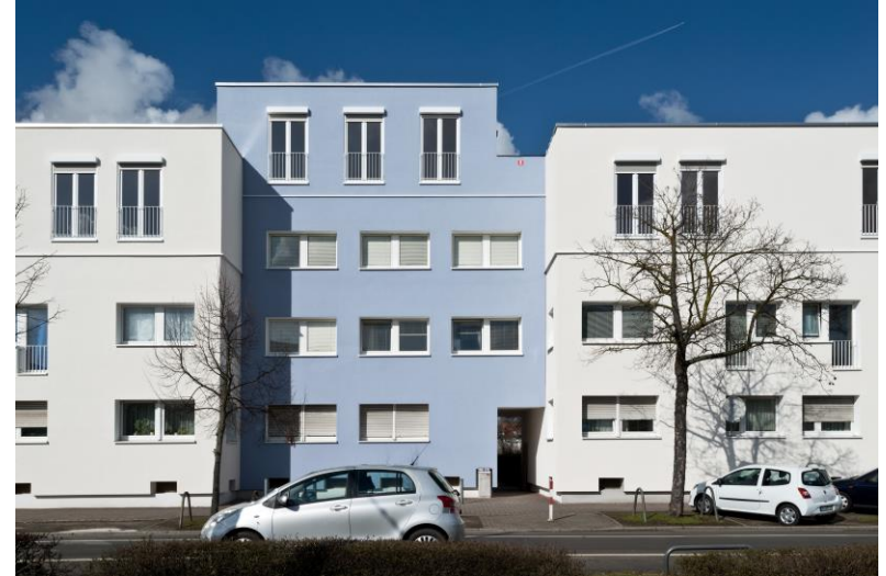
Addition of new floor plus modernization investment
